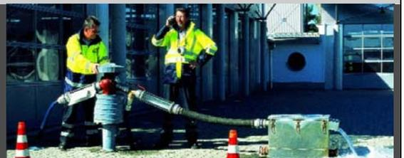
> All moveable sediments are flushed out. Of course without the use of chemicals, without burdening the pipe system through an increased pressure. That is now decisively better than with the common methods. Our impulse flushing method works with a considerably increased degree of efficiency. It cleans more gently, more thoroughly and more sustainably. Which clearly extends the necessary flushing interval. And thus helps save money and inconvenience. >
