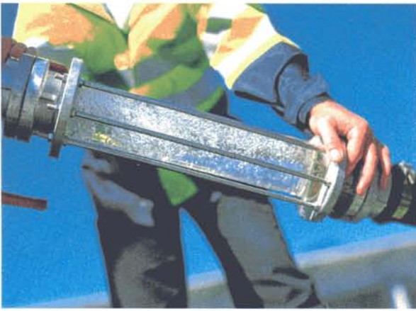
Fig. 2. Complex – An effective way to clean pipelines without chemicals.
