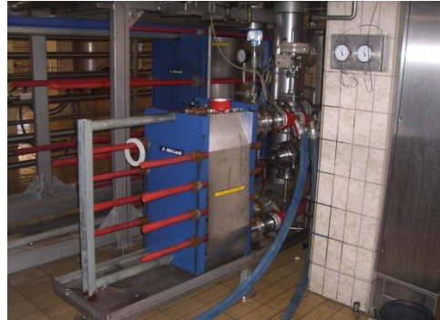
Figure 1: Plate heat exchanger
