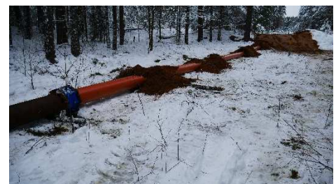
Figure 4: temporary pipeline for discharge
