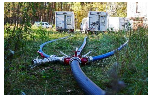
Figure 3: synchronised injection using adapter connections
