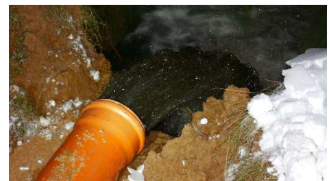
Figure 5: flushing water with mobilised deposits at discharge point
