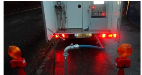
Figure 2: injection using hydrant and stand pipe
