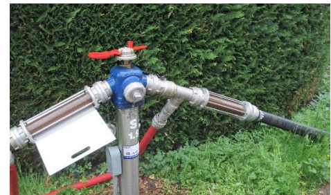
Figure 3: discharge using hydrant with inspection glasses
