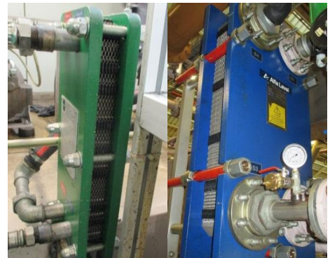
Figure 2: plate heat exchangers in cooling system
