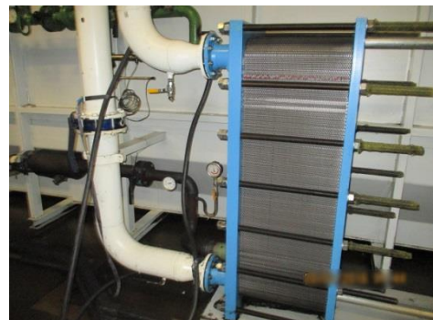
Figure 3: heat exchanger during cleaning
