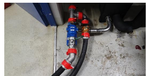
Figure 4: adapters for supply of air and water
