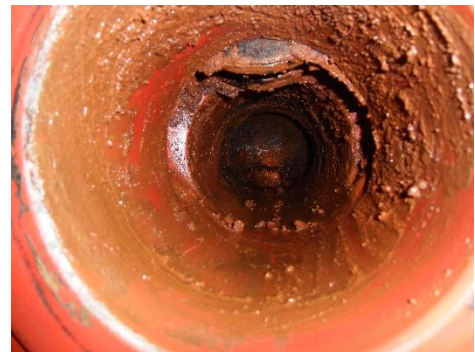
Figure 3: Condition of pipe post -cleaning
