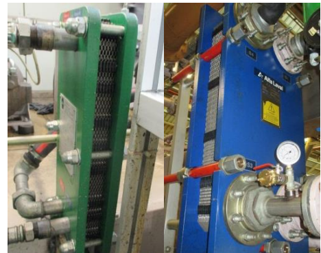
Figure 2: plate heat exchangers in cooling system
