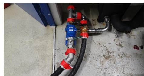
Figure 4: adapters for supply of air and water
