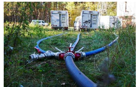
Figure 3: synchronised injection using adapter connections
