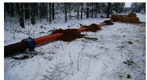
Figure 4: temporary pipeline for discharge
