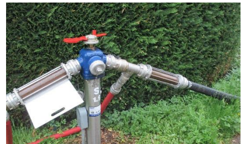
Figure 3: discharge using hydrant with inspection glasses
