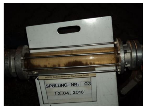
Figure 4: Inspection glass at discharge location
