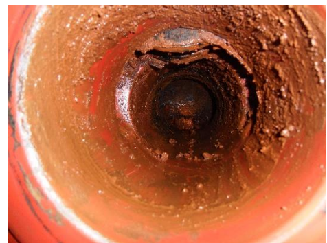
Figure 3: Condition of pipe post -cleaning
