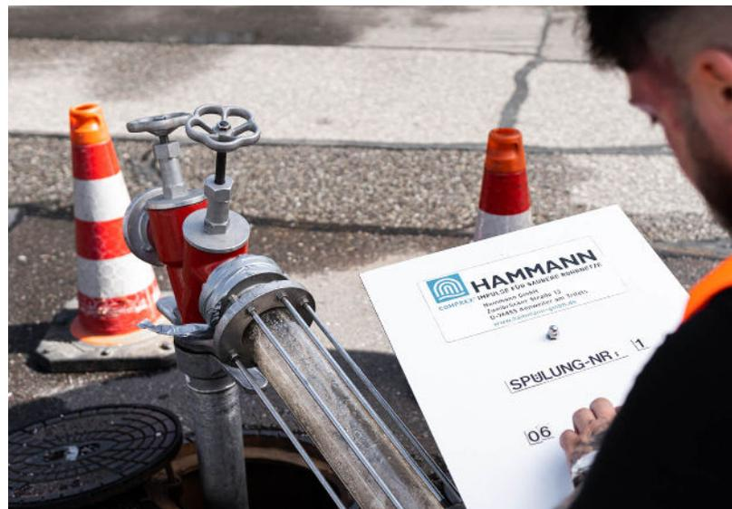
The impulses generate **enormous turbulence** with strong shear and drag forces, whereby they manage to mobilize and reliably discharge existing deposits. The result: clean pipes and clean water – **efficient, gentle** and **economical**.
