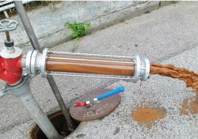
complex® impulse cleaning technology works entirely without chemicals, using **just air and water** according to a principle of physics. We inject filtered air into the section to be cleaned – in a controlled and pulsed manner. This creates packets of air and water that flow through the section at **high velocity**.
