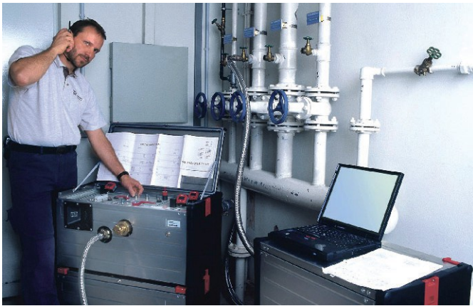
Picture 2 Connecting the pulse flush box to a riser pipe
