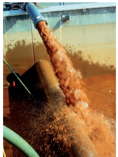
Figure 7: Iron sludge, discharge from well pipe during Complex cleaning Fig. 7: Iron sludge, carried over from a well line, and following separation of flushing water
