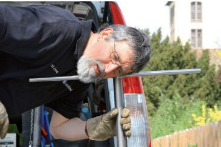
Fig. 1: Listening to a gate valve
