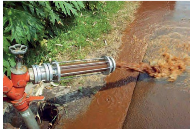
Figure 5: Net cleaning with the Complex process. The detached biofilms stain the rinsing water intensively. At the same time, the animals are also removed - sometimes with thousands of individuals per cubic meter of rinsing water.
