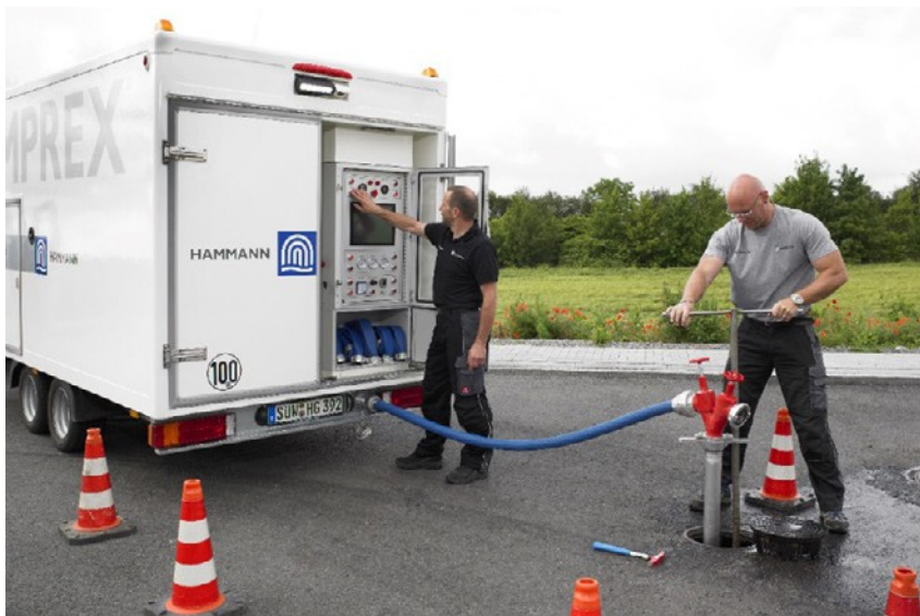
Figure 1: Conventional Comprex unit for flushing the pipe network
