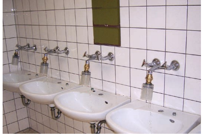
Tapping points with centrifugal separators.
