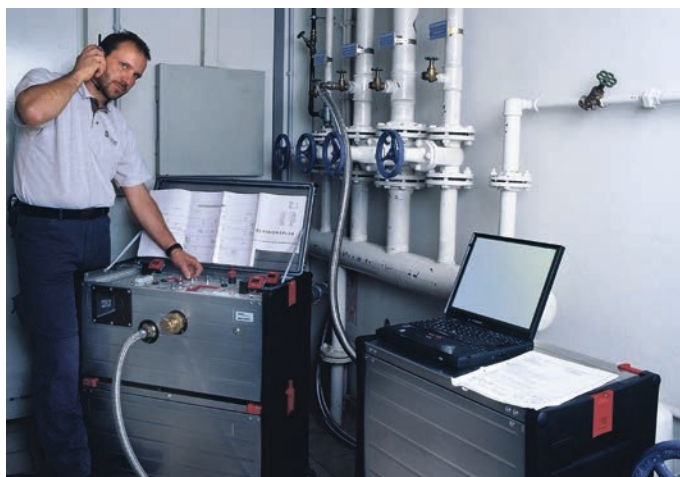
Compressed air supply to distributor.
