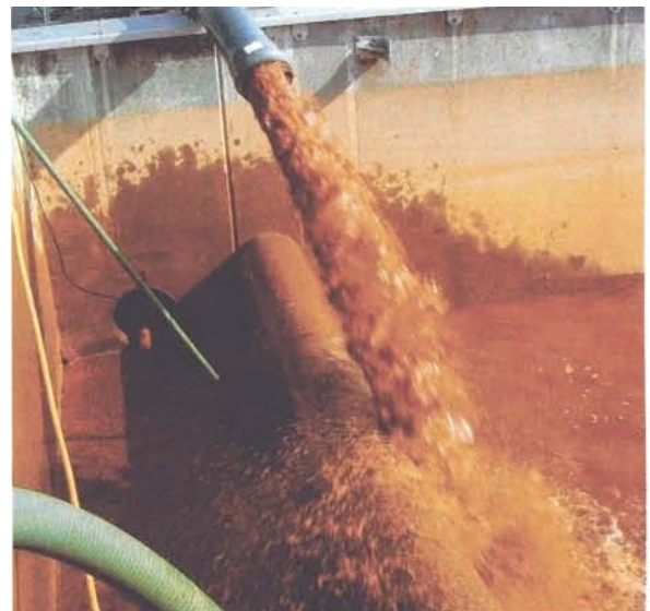
Fig. 1: Removal of ferrous deposits from untreated water pipes in Cham using Complex-VeJahren
