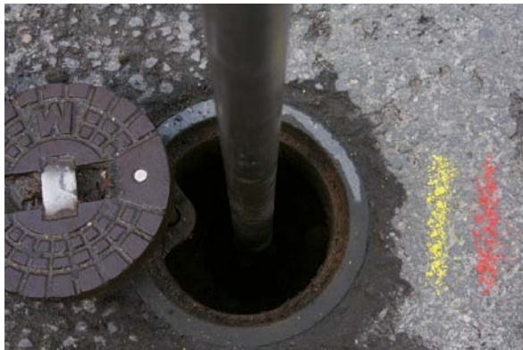
Figure 4: Marking on penalty cap after inspection
