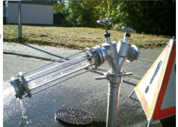
Fig. 2: Water quantity at the feed hydrant shows the slider function: Increased water leakage (top) - poorly closing; low water leakage (bottom) - sufficiently closing
