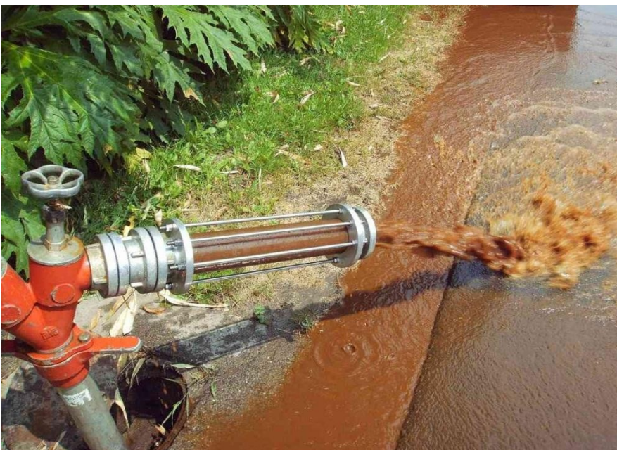
Figure 2: Discharge of deposits during the pulse flushing process
