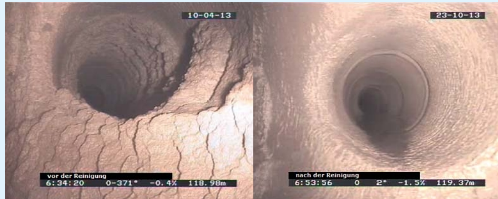
Figure 8 Effectiveness of Complex cleaning on DN 200 well connection pipes Photo:
