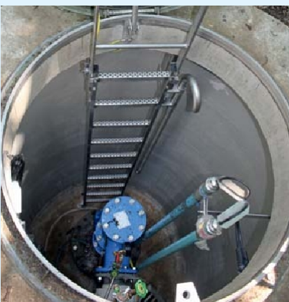
Image 1 Vertical wells on the island of Baumwerder supply the raw water for the Tegel waterworks Photo:
