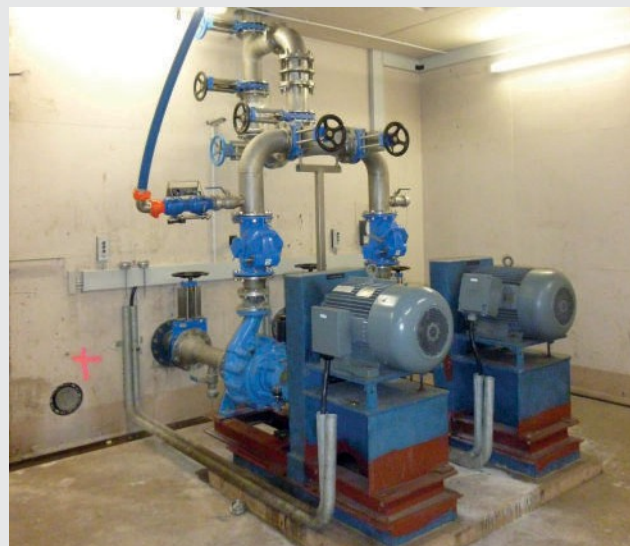
Figure 5: Feed point via pump
