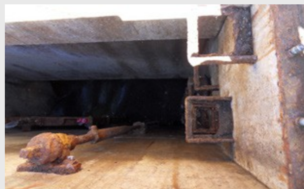
Figure 5: Opened main shaft of the outlet structure with access and additional round closed shaft cover
