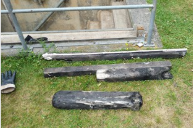
Figure 6: Discharged wooden parts at the entrance to the outlet structure
