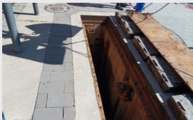
Figure 5: Opened main shaft of the outlet structure with access and additional round closed shaft cover
