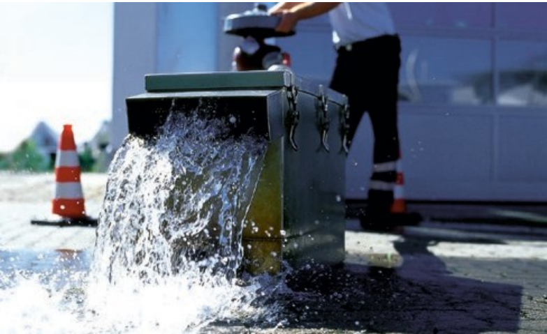
Fig. 2 - Flush box at the outlet point
