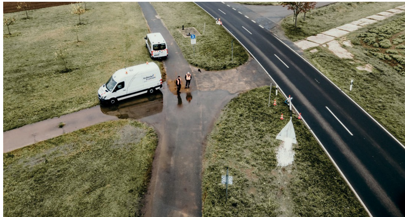
Figure 4 Cleaning a transport line Source: Hammann GmbH
