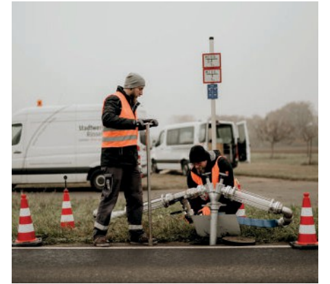
Figure 5 Technicians and equipment at the exit point Source: Hammann GmbH
