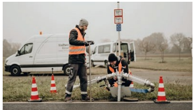
Fig. 2 - Use of the pulse flushing process with compressed air dosing (top) and discharge point (bottom)
