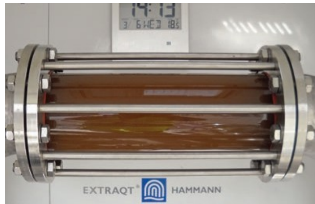
Fig. 5 - Turbidity during water suction flushing as an indicator of hotspots in the drinking water network
