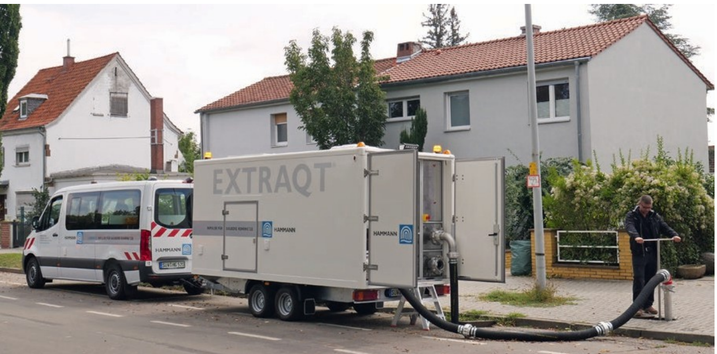
Fig. 4 - Water suction flush in use
