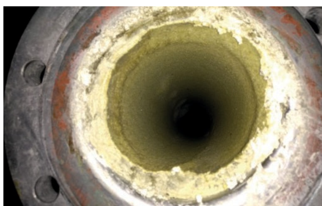
Figure 3: Deposits in the sludge pipe of a wastewater treatment plant and stationary Complex system
