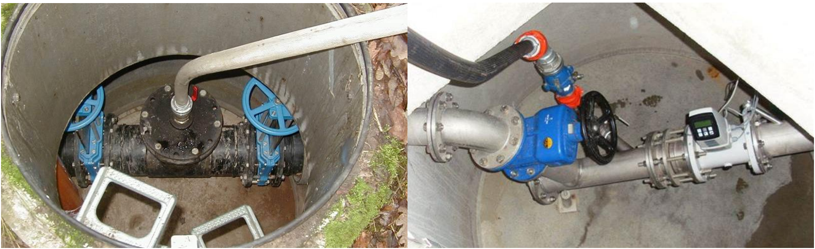
Figure 6: Inlet points for compressed air in wastewater pressure lines at air valve or drain points
